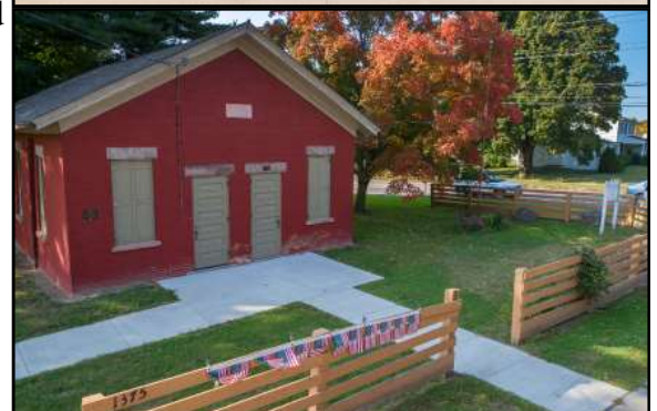
Examples of designated historic districts (Four Corners) and local landmark buildings (Daytons Corner School House).
